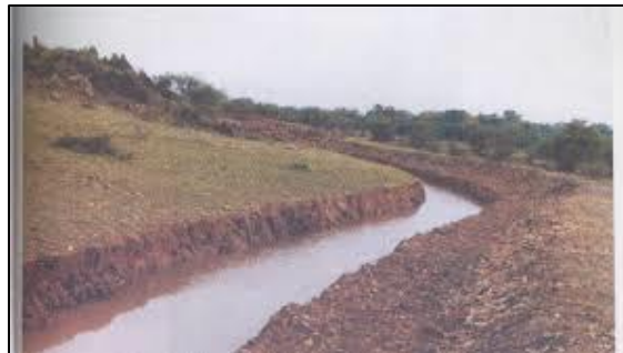
Fig. 6. Placement of Bunding in hilly areas to reduce water flow.
