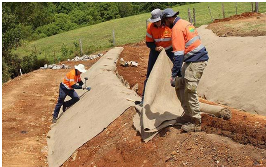
Fig. 4. Use of Mulch sheet on the surface of hilly portion
